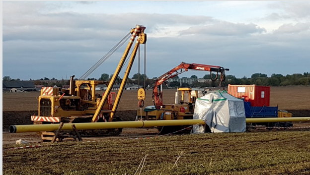
Figure 5: Construction site set-up
