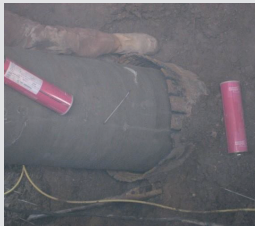
Figure 2: Pulling in a DN 500 water pipe string
